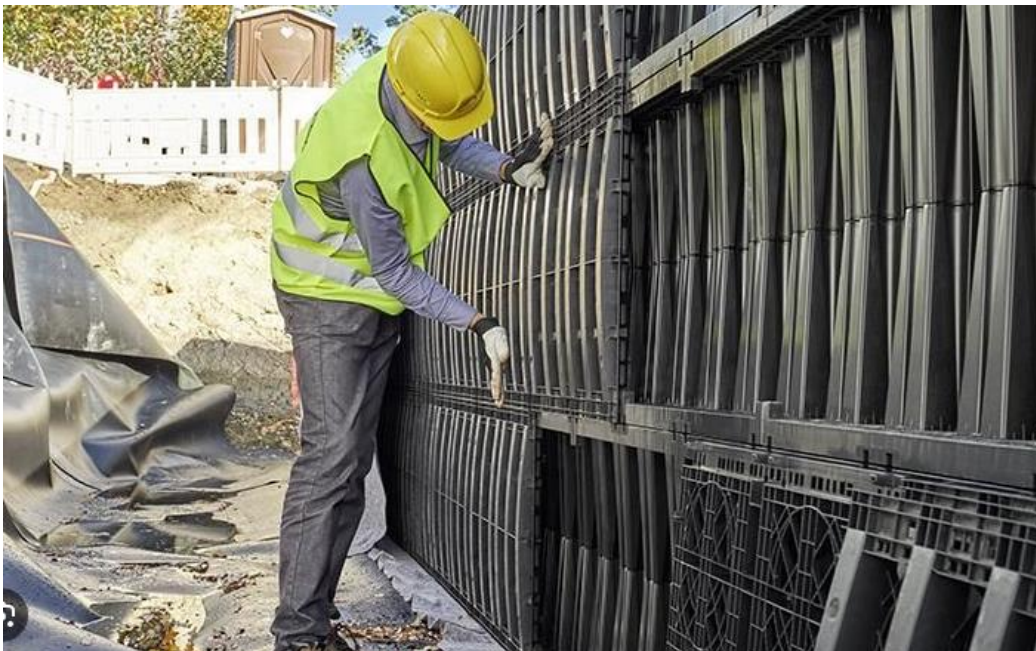
Figure 3.4 Stormbloc Installation
